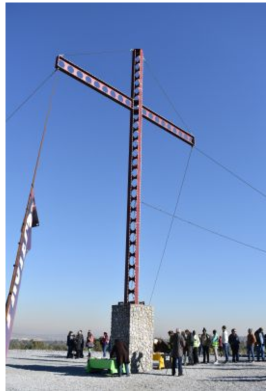
The 18m, illuminated cross boldly shines the love of Christ over the N1 in Tshwane.
