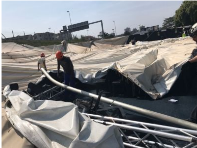
Clean-up crew members removing the flattened DCC tent this week.
